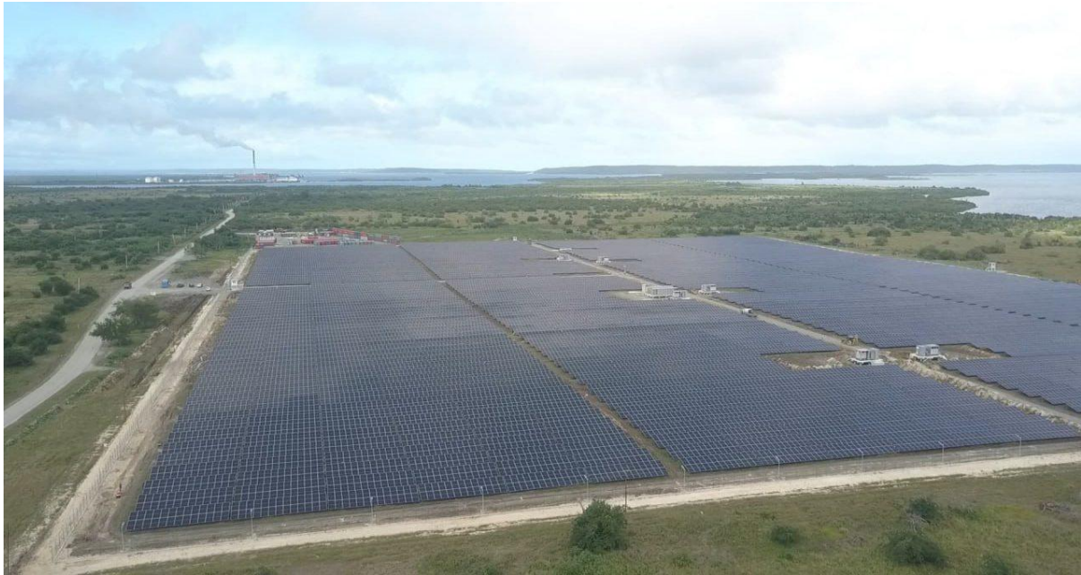
The Corua 5 solar park under construction near Mayarí in the eastern province of Santiago de Cuba (Source: Cubadebate )
